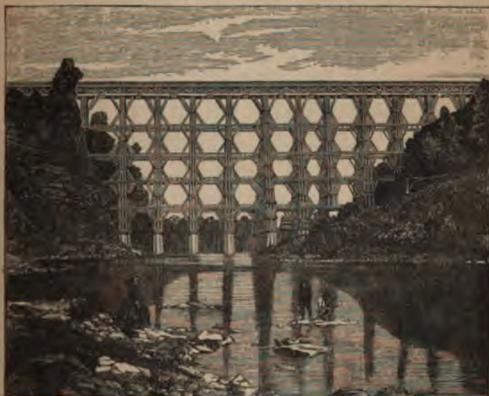
Fig. 220.—[Portage Bridge over the Genesee River, from a Photograph.]
